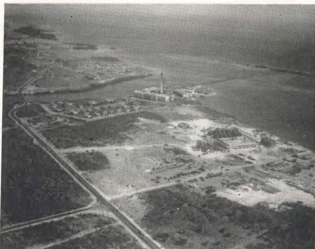
World's largest water distilling plant under construction in Aruba.
